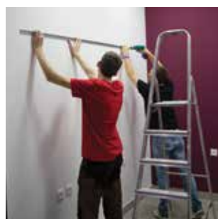
PHASE 1 Installation of the aluminium rail. Installation sur le rail en aluminium.
